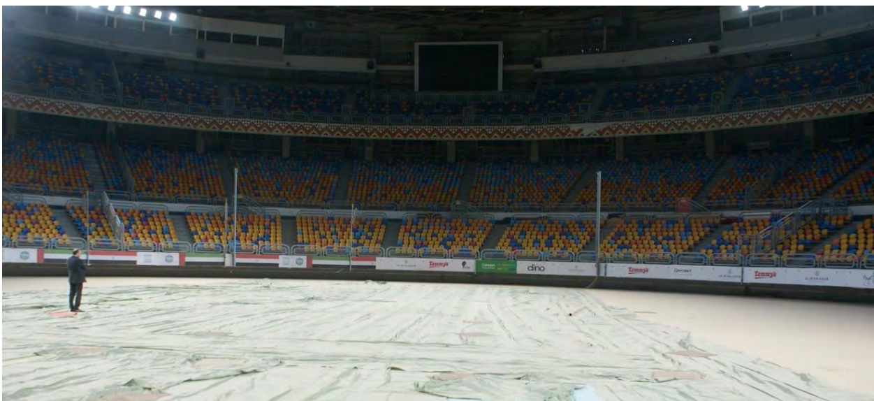
The huge Main Hall, currently under maintenance. Mr. Elhusseiny on the left gives the scale
