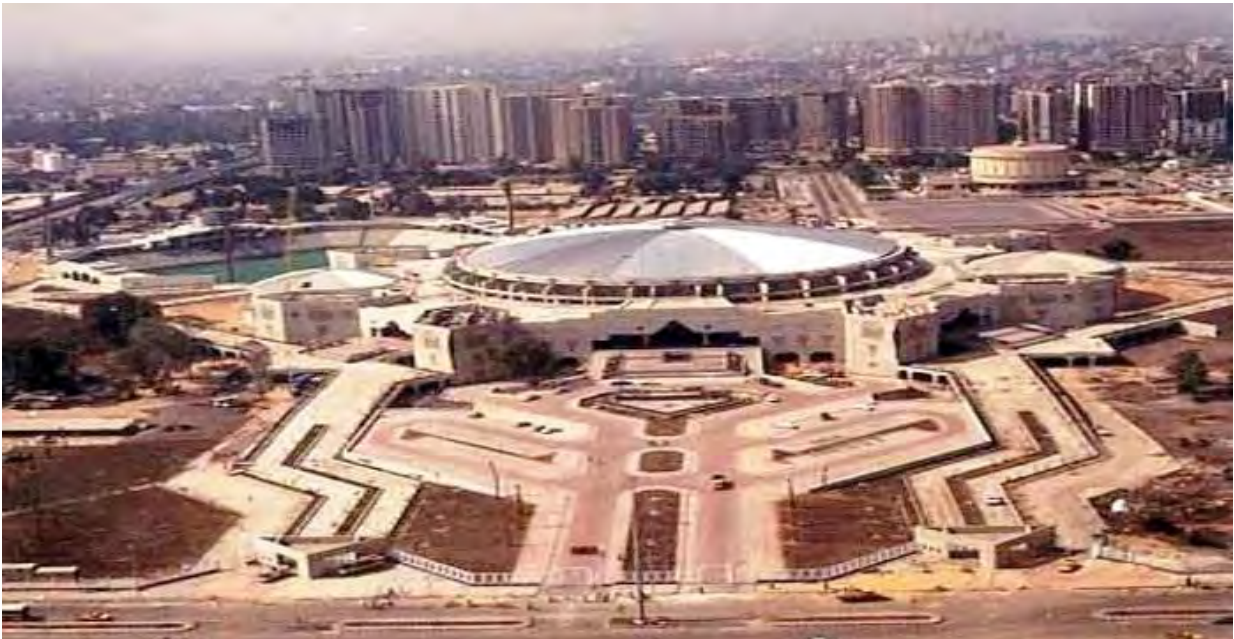
The Cairo Stadium Indoor Halls Complex (Photo from Internet)
